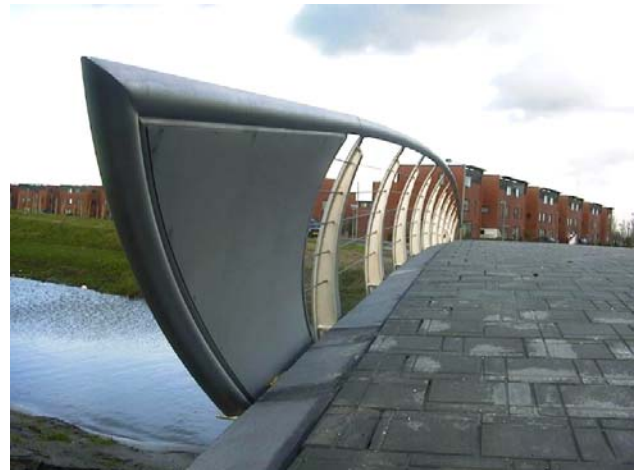
Ceramic blasting of stainless steel bridge parts
